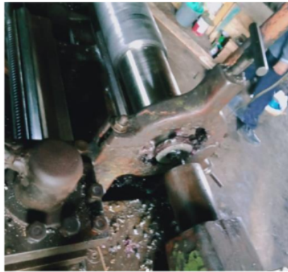
Gambar 33. Proses pelubangan as mesin press
