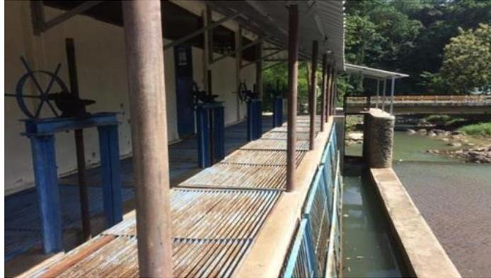
Gambar 2. Intake Gravitasi
