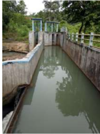
Gambar 2. Intake Gravitasi
