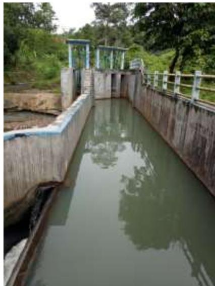
Gambar 2. Intake Gravitasi
